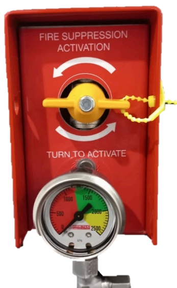
Manual actuator with anti-tamper tie
